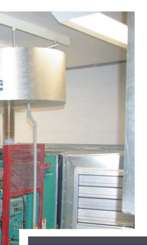
Significant noise reduction measures were required to achieve the limits. A two-stage noise reduction system was deployed including acoustic louvers and acoustic duct silencers on the intake and outlet ducts used to keep the generator cool while in operation. The generator exhaust includes a dual-stage silencer.
