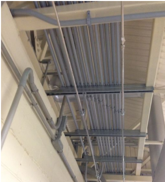
New conduits to route control systems back to the RPU.
